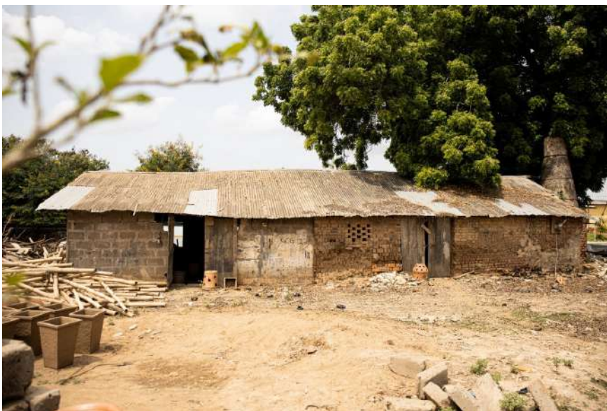
Figure 4: The structure built by Michael Cardew in Vume for Women to practice pottery
